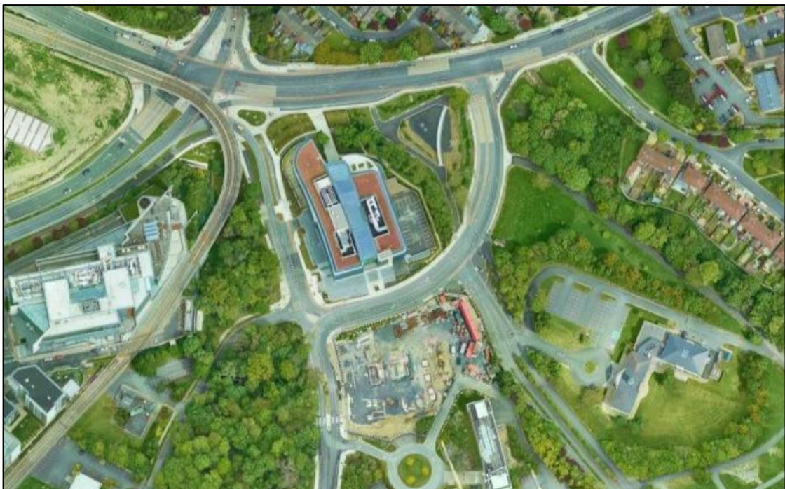
Figure 2.6: Aerial view of the Mastercard Innovation Campus, South County Business Park, Leopardstown, Co. Dublin, showing Phase 1 of construction completed and Phase 2 under construction. (Source: Google Earth.)
