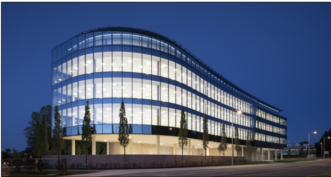
Figure 2.4: Mastercard Innovation Campus, South County Business Park, Leopardstown, Co. Dublin. (Source: Cyril McGuire.)
