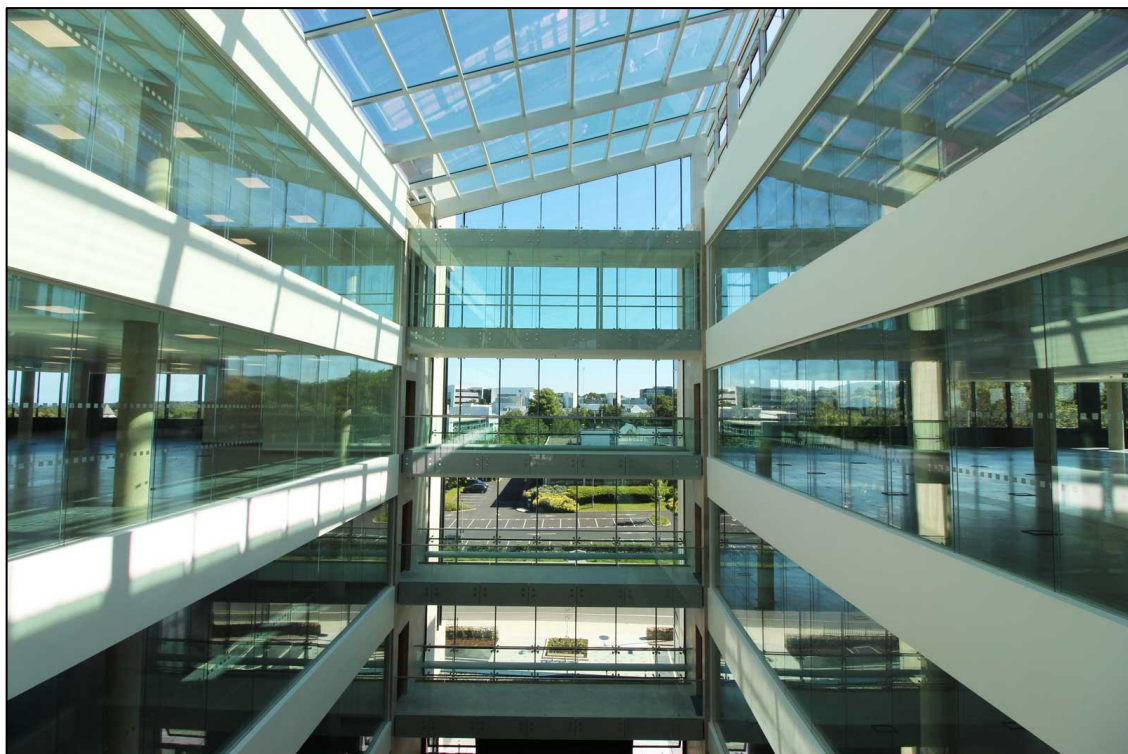
Figure 2.2: Mastercard Innovation Campus, South County Business Park, Leopardstown, Co. Dublin. (Source: Mastercard.)
